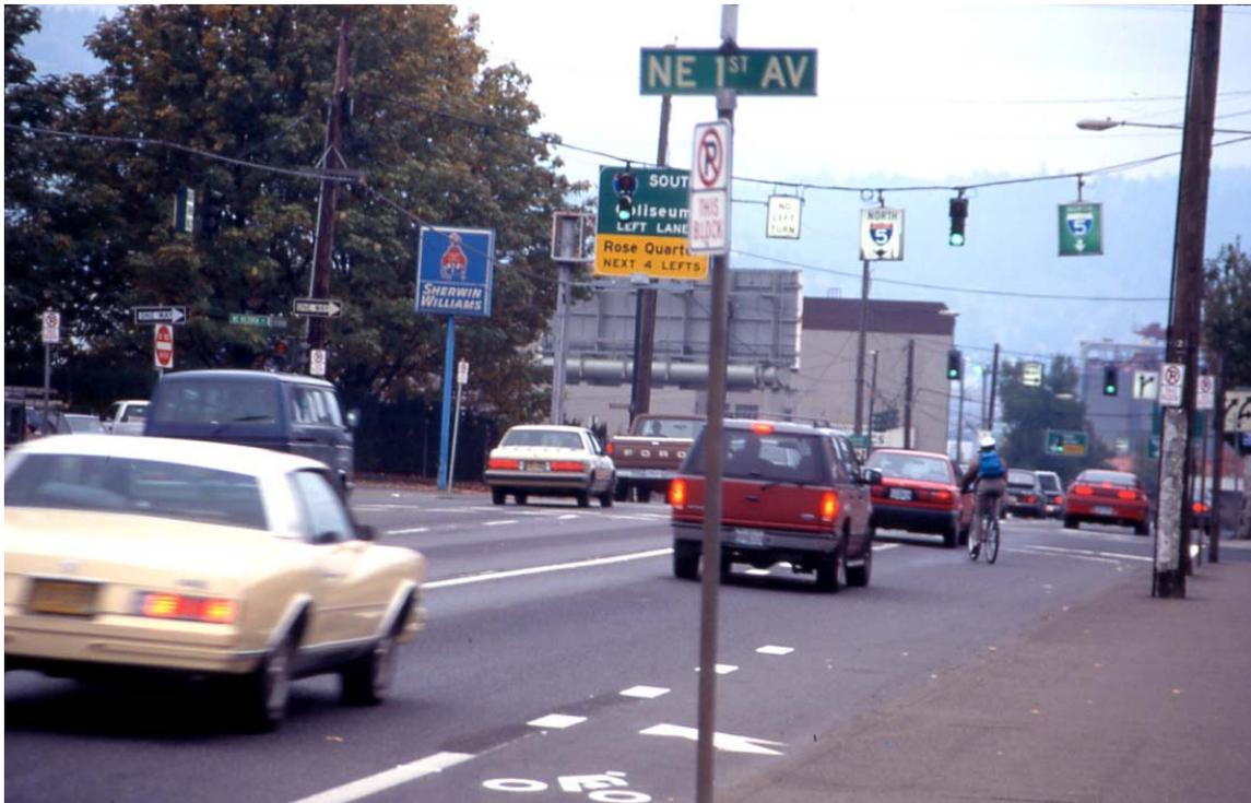
This photo illustrates an abrupt end of the bicycle facility. This is a hazard for the cyclist and motorist, because it forces the cyclist to merge abruptly into dense traffic.
